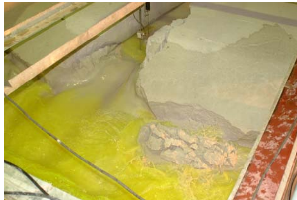
Figure 2-14. Notching and sediment slump in washover throat and sediment slump on dune face.
