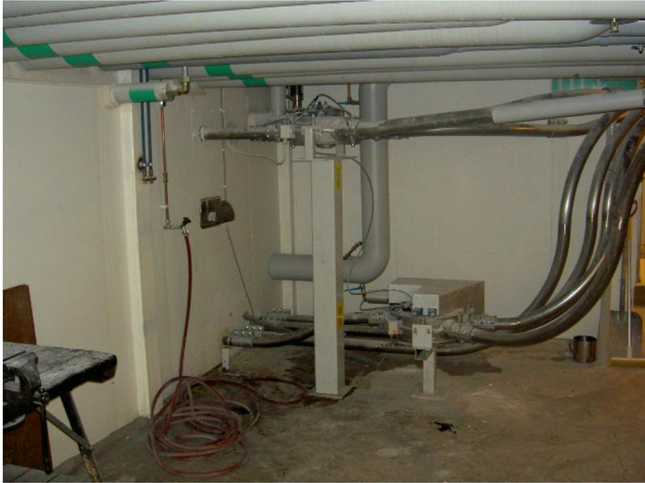
Figure 6, Pneumatic conveying pipes in the attic
