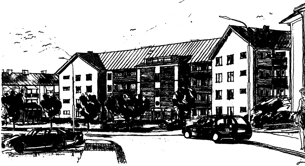
Figure C.1 An overview of the multi-storey apartment building Orgelbänken. Orgelbänken consists of a single building with four floors and an attic. Wood-panel is the facade material in access balconies and in stairwells and plaster in the rest of the building. [40]
