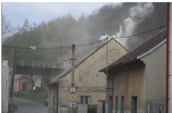
A building in Zákolany using coal for heating
