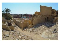
Figure 1.5 Deterioration of vernacular houses and replacement with concrete skeleton ones in the Farafrah oasis.
