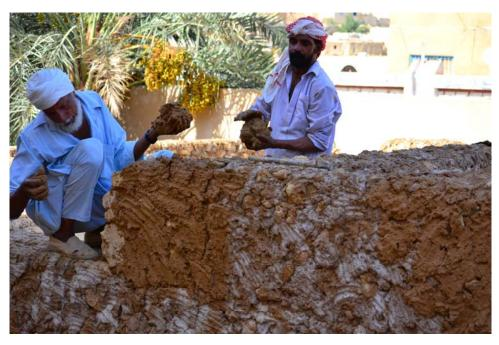
Figure 2.15 Vernacular builders in the Siwa oasis using salt blocks (Karshif) and mud. Roof construction is palm wood and mud brick.
