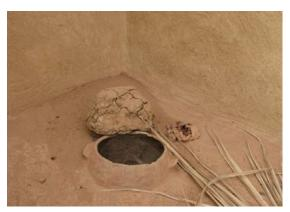
Figure 4.12 Bottomless pottery vessels serve both as skylights and ventilation openings.
