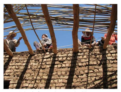
Figure 2.20 Traditional roof structure making process in the Dakhla oasis.
