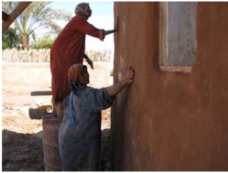
Figure 5.32 Exterior wall rendering with the help of Balat ladies using traditional manual techniques.
