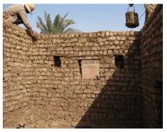
Figure 5.24 Windows and niches during wall construction.
