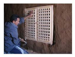
Figure 5.36 Local carpenter while hanging the cabinet door inside the room.
