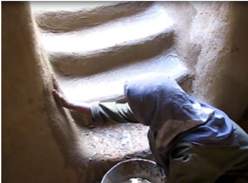
Figure 2.37 Monthly plastering maintenance for houses done regularly by women in the Dakhla oasis.
