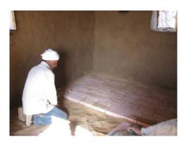
Figure 5.34 Floor making using sand tiles.
