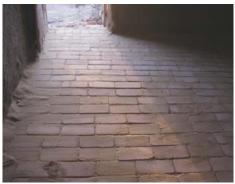
Figure 5.35 Sand floor tiles after finishing.
