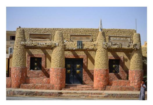
Figure 2.16 Local bank branch designed and constructed by The Siwa Sustainable Development Initiative with earth vernacular building technology in the Siwa oasis using Karshif. According to the designer, the building passed safety and security bank tests in 2008.
