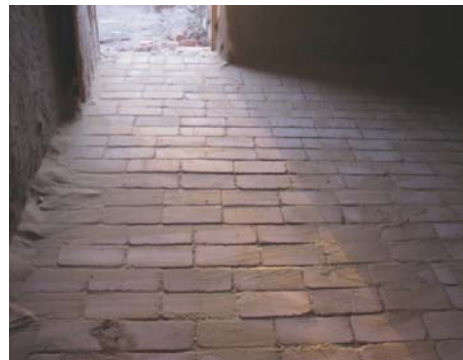
Figure 5.35 Sand floor tiles after finishing.
