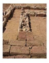
Figure 5.21 The stone and brick footing.
