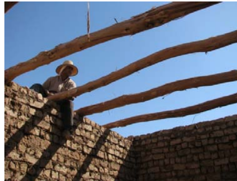
Figure 5.26 Placing the wood logs on the walls.
