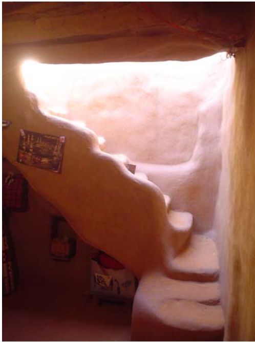
Figure 4.13 Staircase shaft function as wind catchers.
