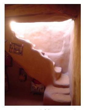
Figure 4.13 Staircase shaft function as wind catchers.
