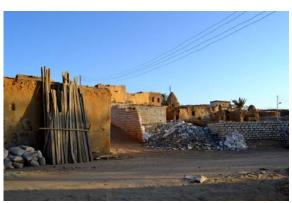
Figure 1.2 Deterioration of vernacular architecture and replacement of vernacular houses with concrete skeleton and white brick ones in the Baharia oasis.
