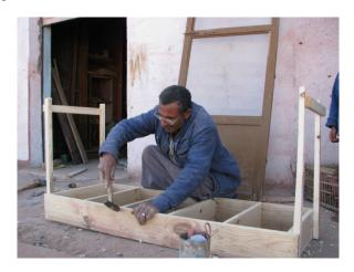
Figure 5.11 Kamel, the local carpenter in Balat, while working on implementing the new mould of size  $50\text{cm} \times 25\text{cm} \times 15\text{cm}$ .
