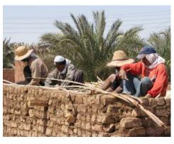
Figure 5.28 Placing palm leaves on top of reeds.
