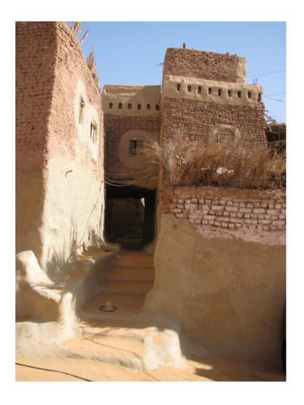
Figure 4.83 Example of a well-maintained semi-private alley with built-in mud brick benches.
