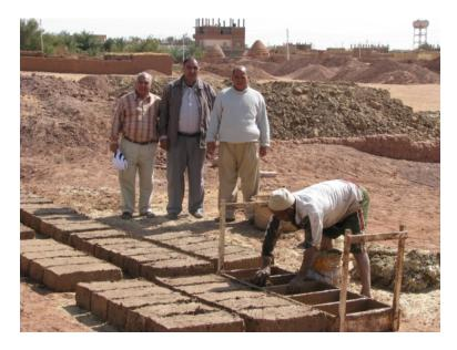
Figure 5.12 Mud brick casting using the first alternative of the mould and the representatives from the local municipality visiting the site to follow the work in process.
