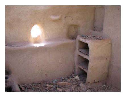
Figure 4.33 Examples of furniture, curved smooth walls, and of an opening made of clay in a deserted house.
