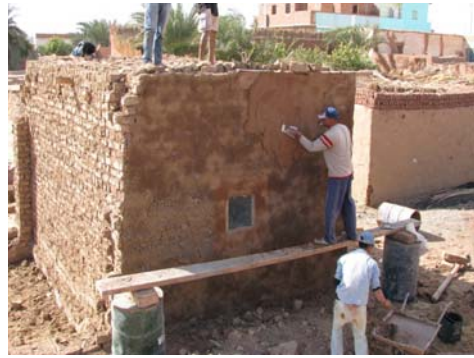
Figure 5.33 Exterior wall rendering using plastering trowels.
