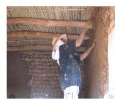
Figure 5.30 Plastering layer is thrown on the walls.
