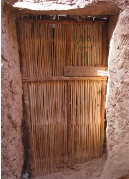
Figure 2.34 Doors in the Dakhla oasis made from palm tree ribs or reeds and the wooden key and lock are made from building construction wood leftovers.
