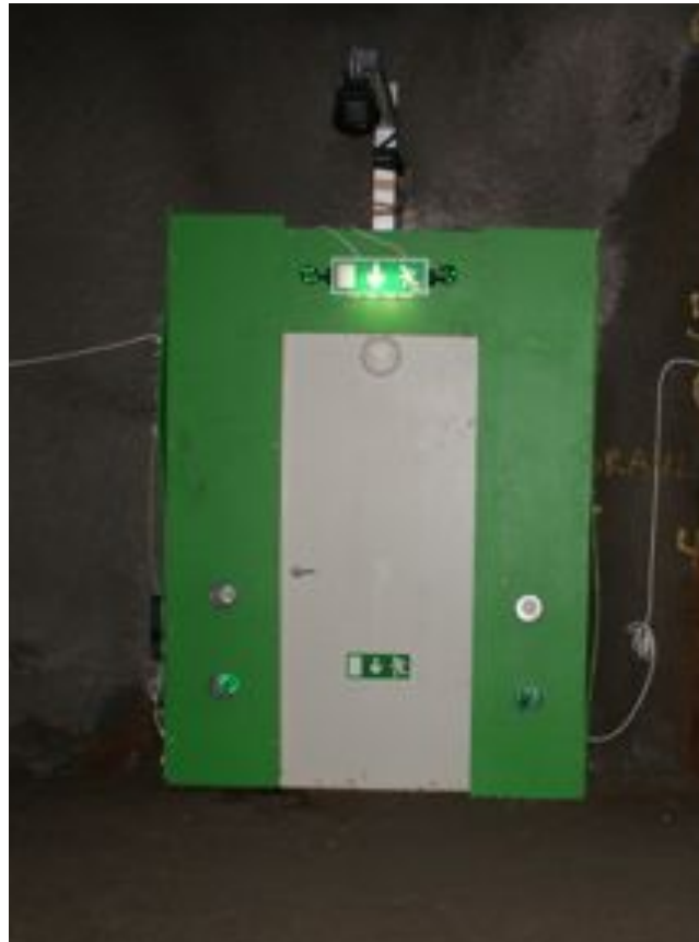
Figure 8. The emergency exit installed on the left side, approximately 180 metres into the tunnel.
