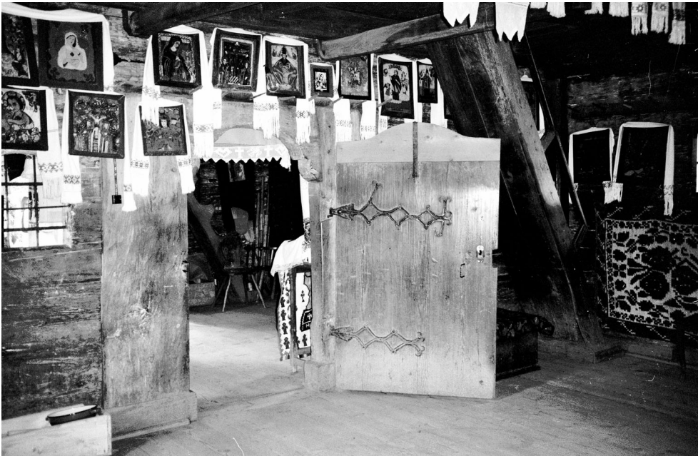
70 Ieud Șes . The decorative iron hinges of the inner door to the nave (below) remind of the surviving hinge from the inner door in the church of Dragomirești (above) indicating the work of a single smith behind both. The two close churches were also built soon one after the other in the 1710s. Photos: July 1997 (below) and June 1999 (above).
