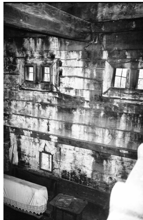
93 Rona de Jos . The cross beam penetrates the interior under the spring of the vault in between the two upper pairs of windows. Photo: October 1997.
