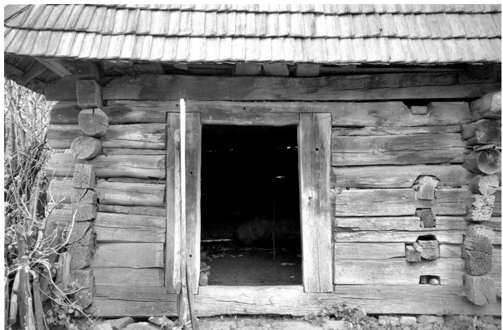
66 Crăcești. The poor stable of Costin Grigore a lu Zaharie retains a simple door sided by jambs and mounted in the sill bellow and a beam above without any tenon. It is hold in place by the slots carved from the sill and the beam above. The lateral grooves receive the tenon of the wall logs. Photo: October 2000.
