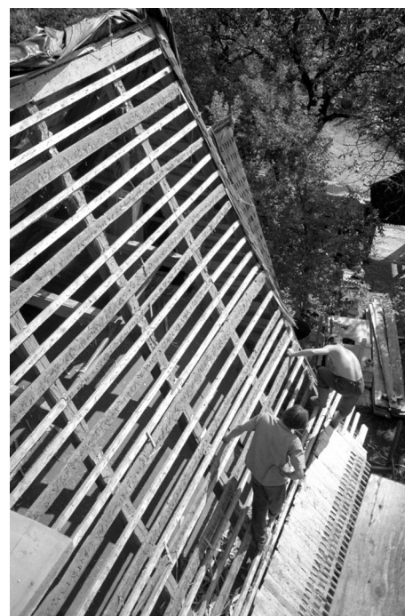
94 Ieud Deal . The old lathing was easily distinguishable by its massive appearance under the repair of the roof. Photo: August 1997.
