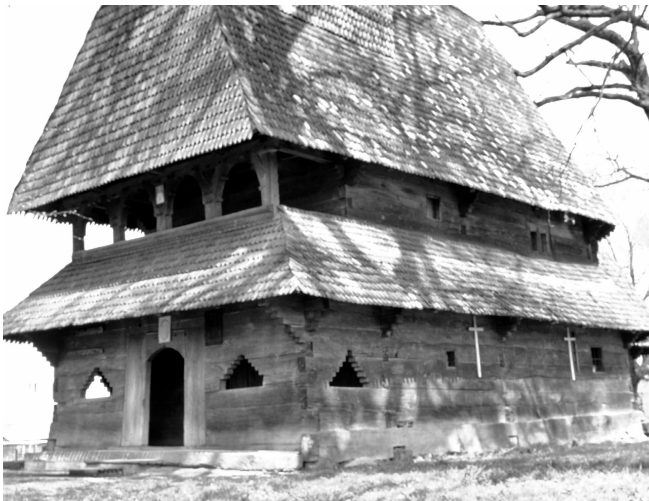
162 Krainykovo. In comparison to the earlier churches with eyes the antechurch was built here from the same wall beams as the rest of the church. Photo: April 2002.
