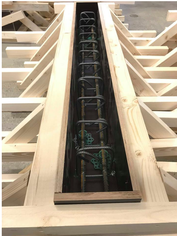
Figure 24: Finished form
