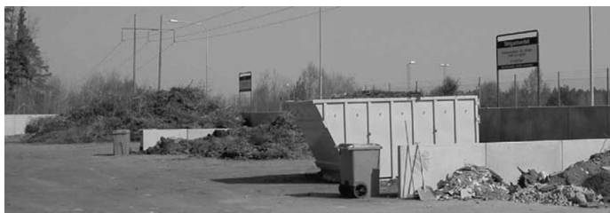
Fig. 4. The dump area for garden waste and excavated materials at Malmen Recycling Centre.
