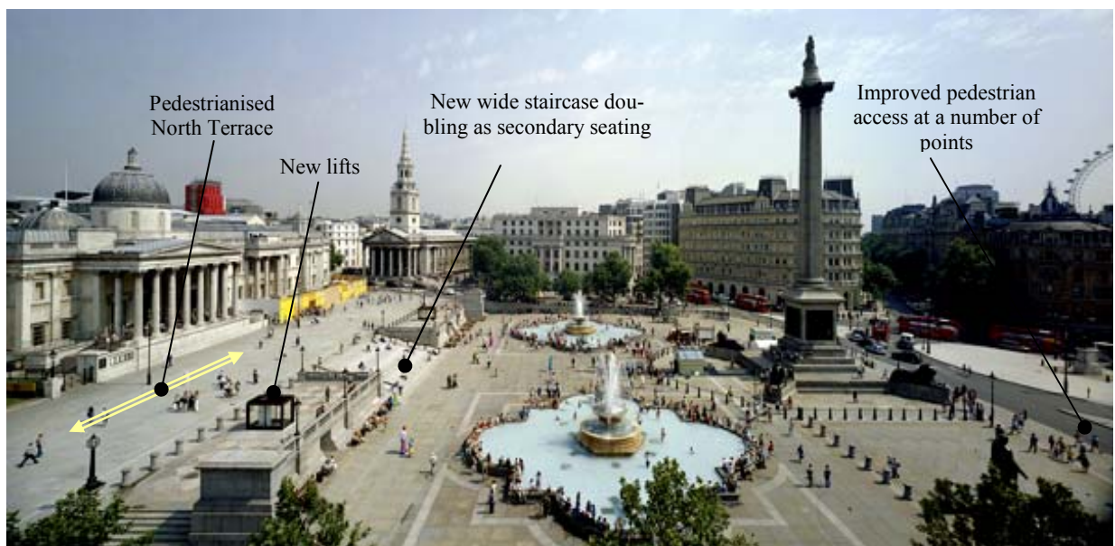
Trafalgar Square after reconstruction – North Terrace was pedestrianised, now acting as better pedestrian link in the area and connecting the National Gallery to Trafalgar Square. The new space reinforces Trafalgar Square's status and value as a 'World Square'.
