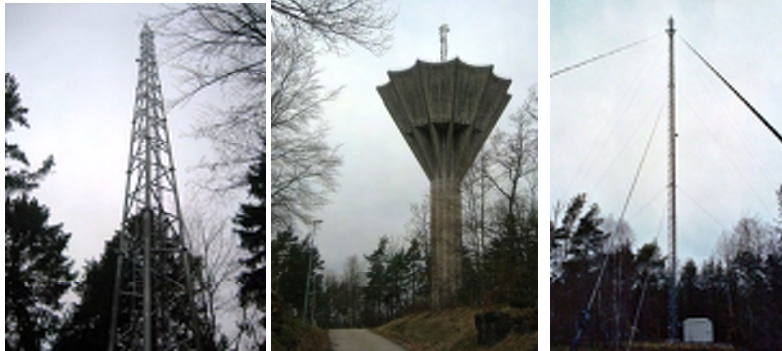
Pictures: To the left, a 3G tower in Gammalstorp, Blekinge. In the middle, a telecom mast on water tower in Bräkne-Hoby, Blekinge. To the right, a mast with tech shed in Äryd, Blekinge.
