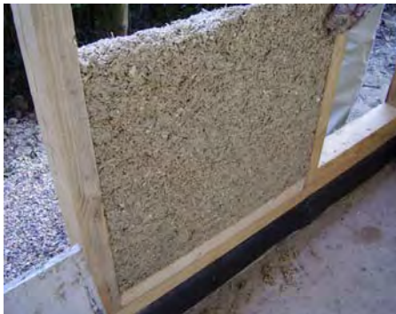
Figure 2. Tamped hemp after the temporary siding has been removed.
