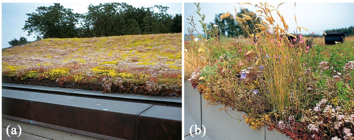
**Figure 3.** Extensive (a) and intensive (b) green roofs. Source: Veg Tech.
