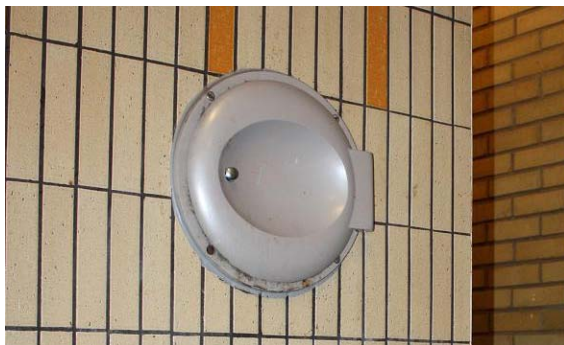
A locked waste chute in Sweden
