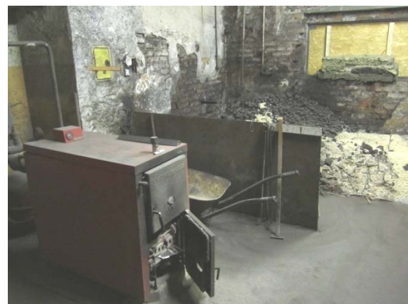
A “dirty” boiler and accompanying coal supply.
