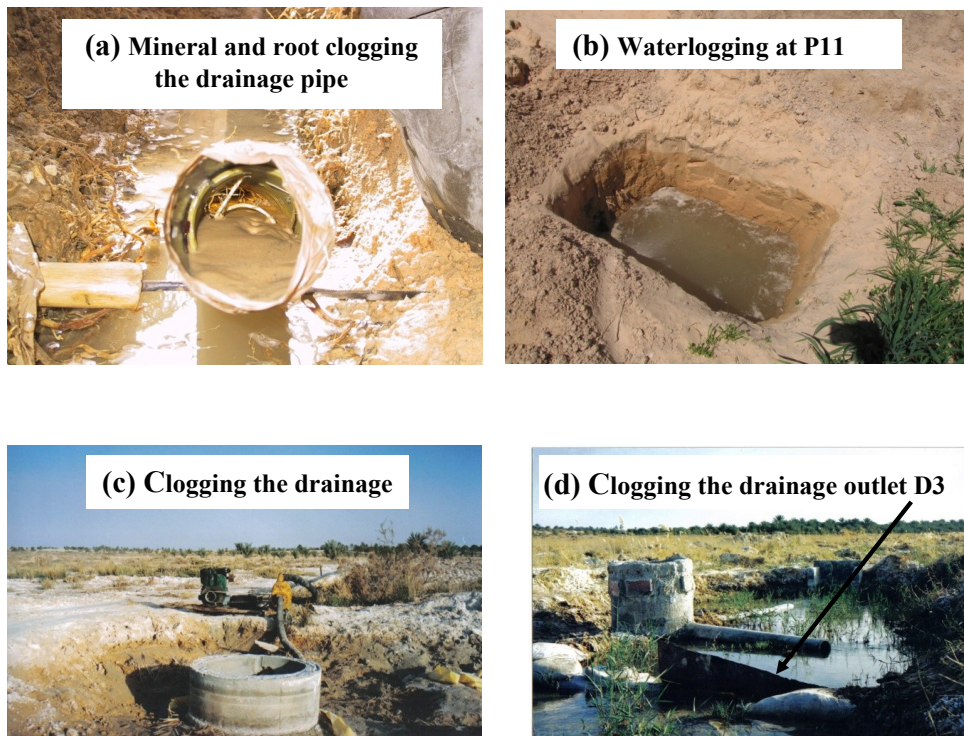
Figure 16. Main causes of the low drainage network efficiency. (a) Mineral and root clogging the drainage pipe, (c, d) irrigation of illegal palm extension by clogging the drainage network.
