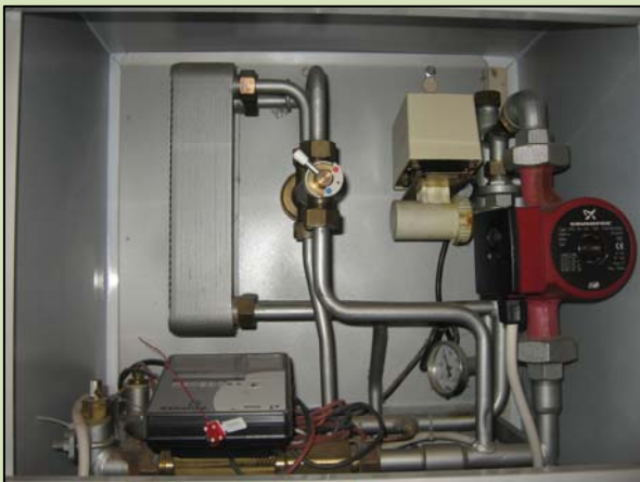
Example of an installed household heat exchanger
