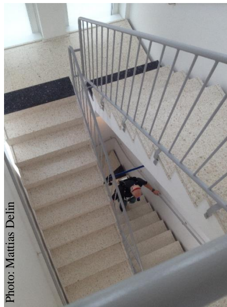
Figure 12. The stairwell in the Ideon experiment.
