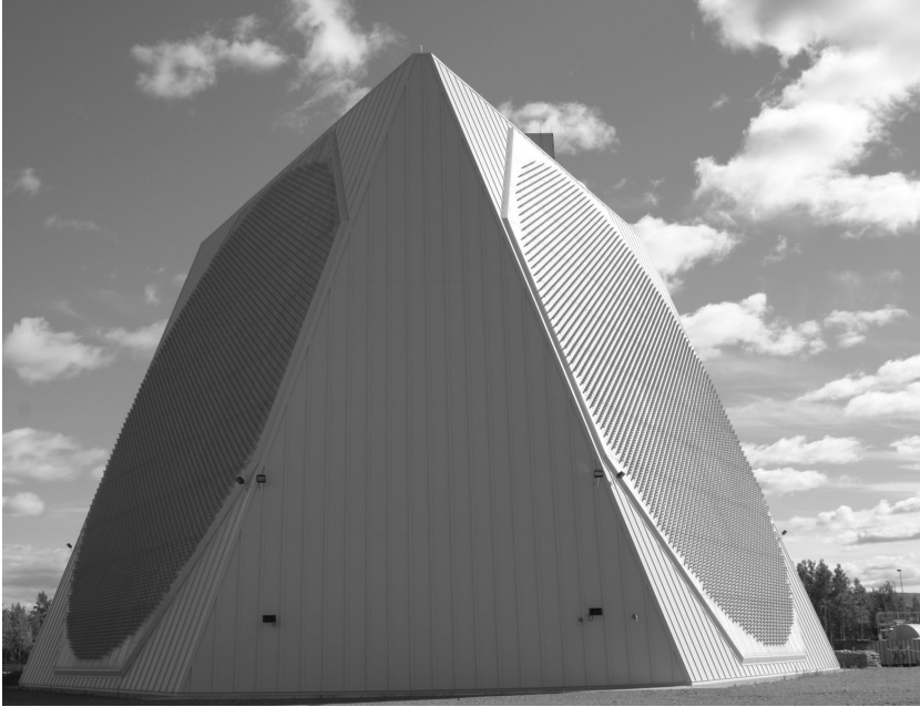
Figure 39: Figure of a phased array. This large, 27 m in diameter, phased array is placed in Alaska to monitor the northern sky as a part of the ballistic missile early warning system. Courtesy of Alaska District
