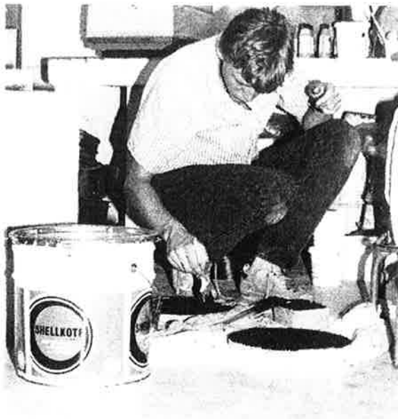
Fig. 6. Painting the bituminous emulsion in proposal 3.
