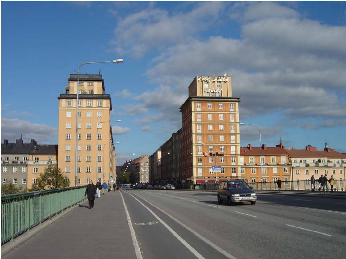
The bridge "St Eriksbron" towards Birkastan
