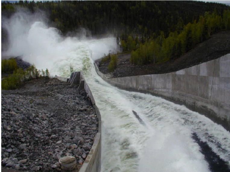
Figure 6-6 – Discharge of water.
