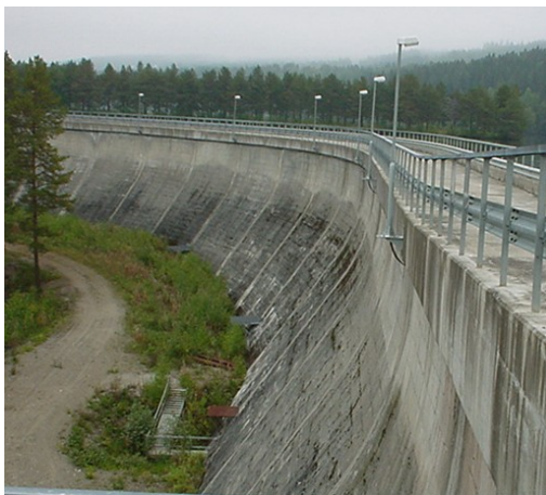
Figure 2-1 - Gravity dam at Stadsforsen.
