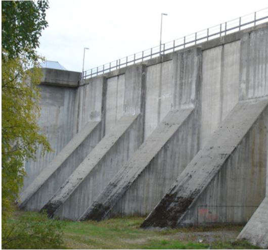
Figure 2-2 - Buttress dam at Stornorrfors.
