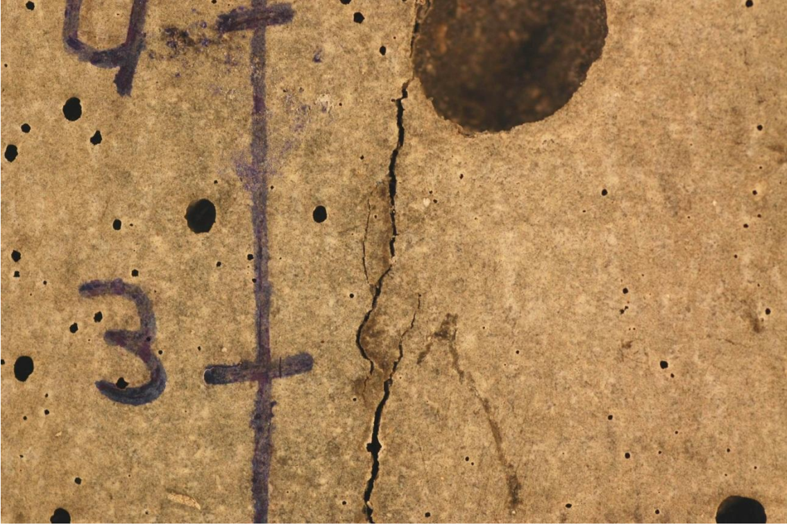
Figure A2.3: 0.2 mm crack after 1 year cyclic immersion in sea water and drying. Test series 1, specimen H75-2-2-1.
