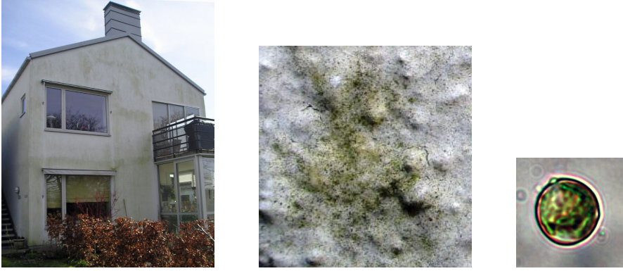
Figure 3.1: Algae growth on a building façade (left), a close up picture (middle) and as seen in microscope (x400) (right).
