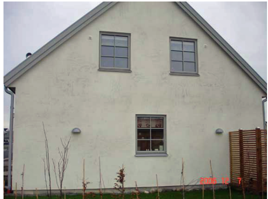
(b) Building with mould growth
