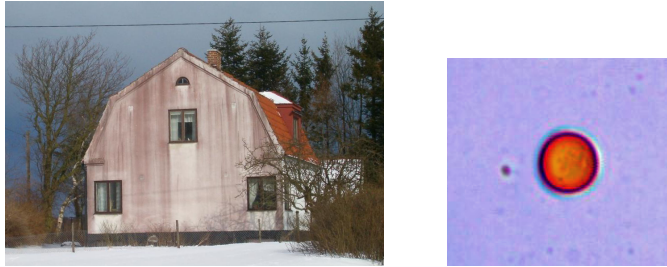
Figure 3.2: Red coloured green-algae ( Haematococcus pluvialis ) on a building façade (left) (photo: L. Wadsö) and as seen in microscope (x400) (right).
