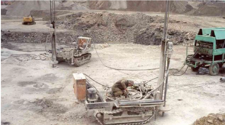
Figure 1.3: The Anelema quarry, Estonia. Photo: Sirkku Holmberg.
