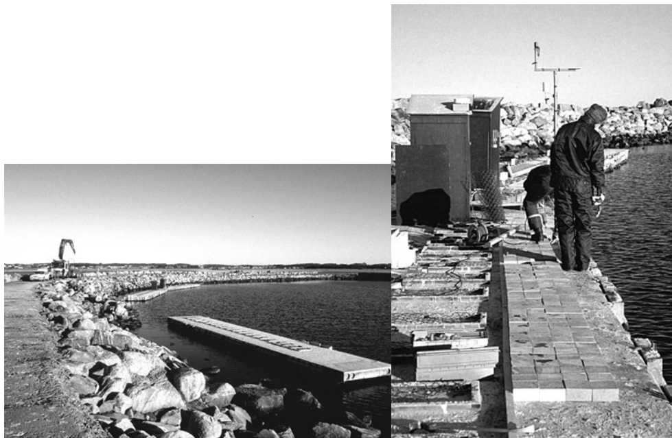
Figure 11.2 Field exposure site in a marine climate at Träslövsläge harbour. Specimens are mounted on top of pontoons.
