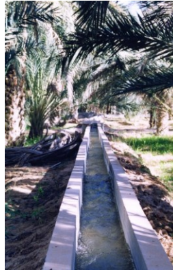
After : Open concrete channels
