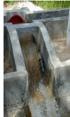
After : Open concrete channels
