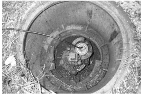
Figure A.6: Connected fire hydrant cap with incorporated transducer.
