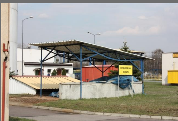
CLEANING FACILITY FOR RAW BIOGAS
