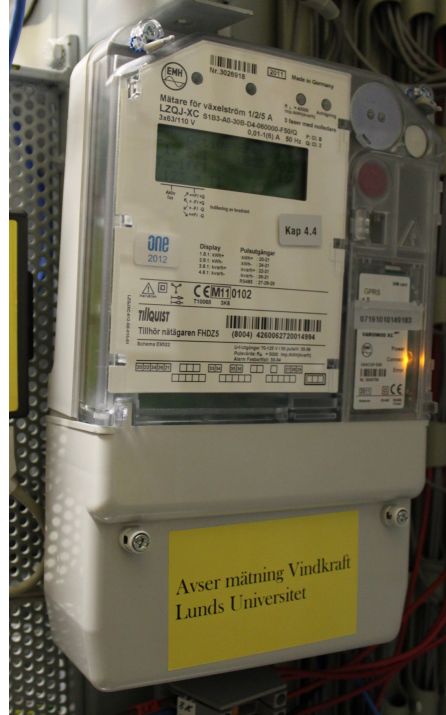
Figure 5.5: Electricity meter of type EMH LZQJ-XC which is mainly used in the field test.
