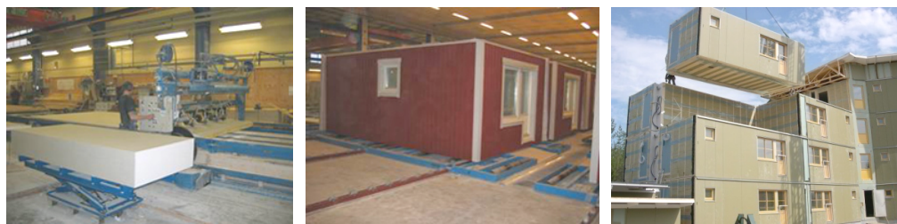
FIG 2: Modular house production
