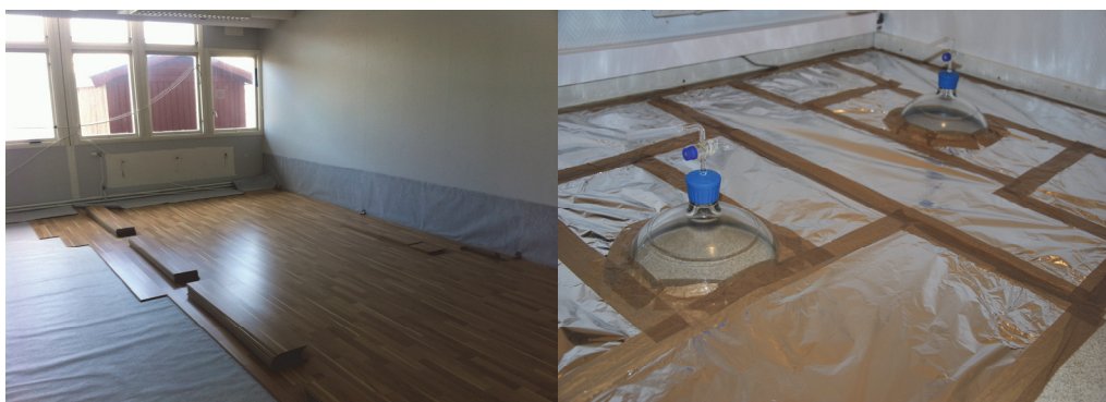
Picture 1. Installation of the cTrap above the source of emissions in a school building (left) and an office room (right, courtesy Jörgen Grantén, Lund, Sweden).
