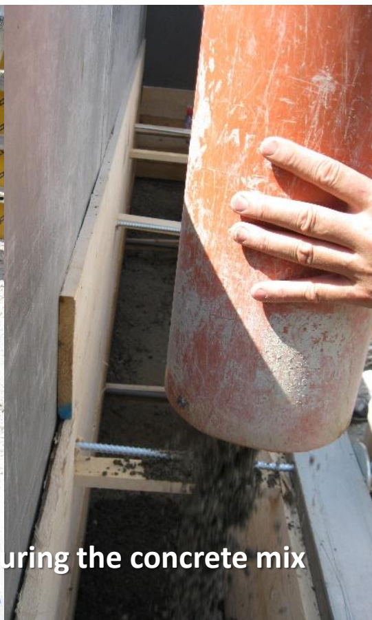
Foundation formwork assembly
