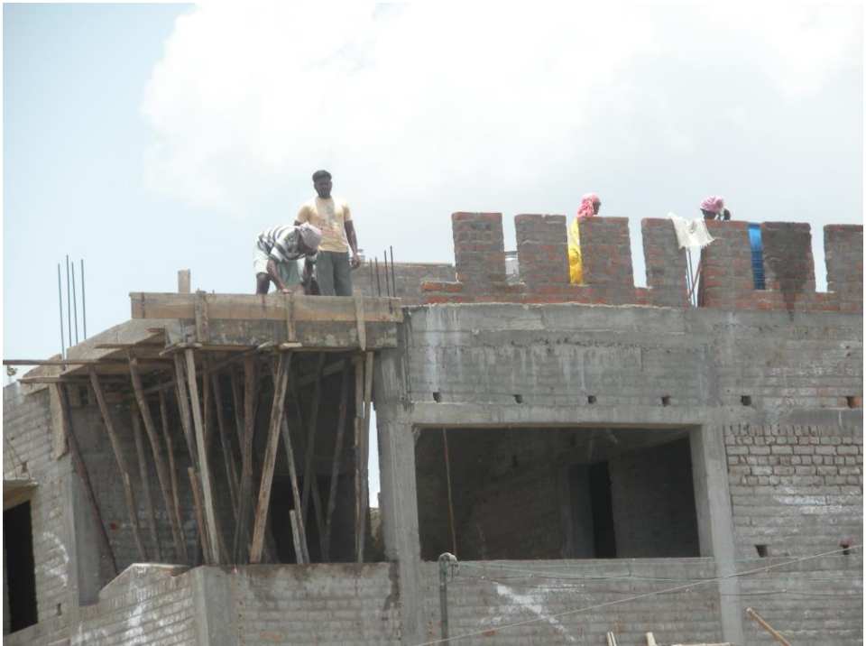
Figure 12: Picture from the construction site.
