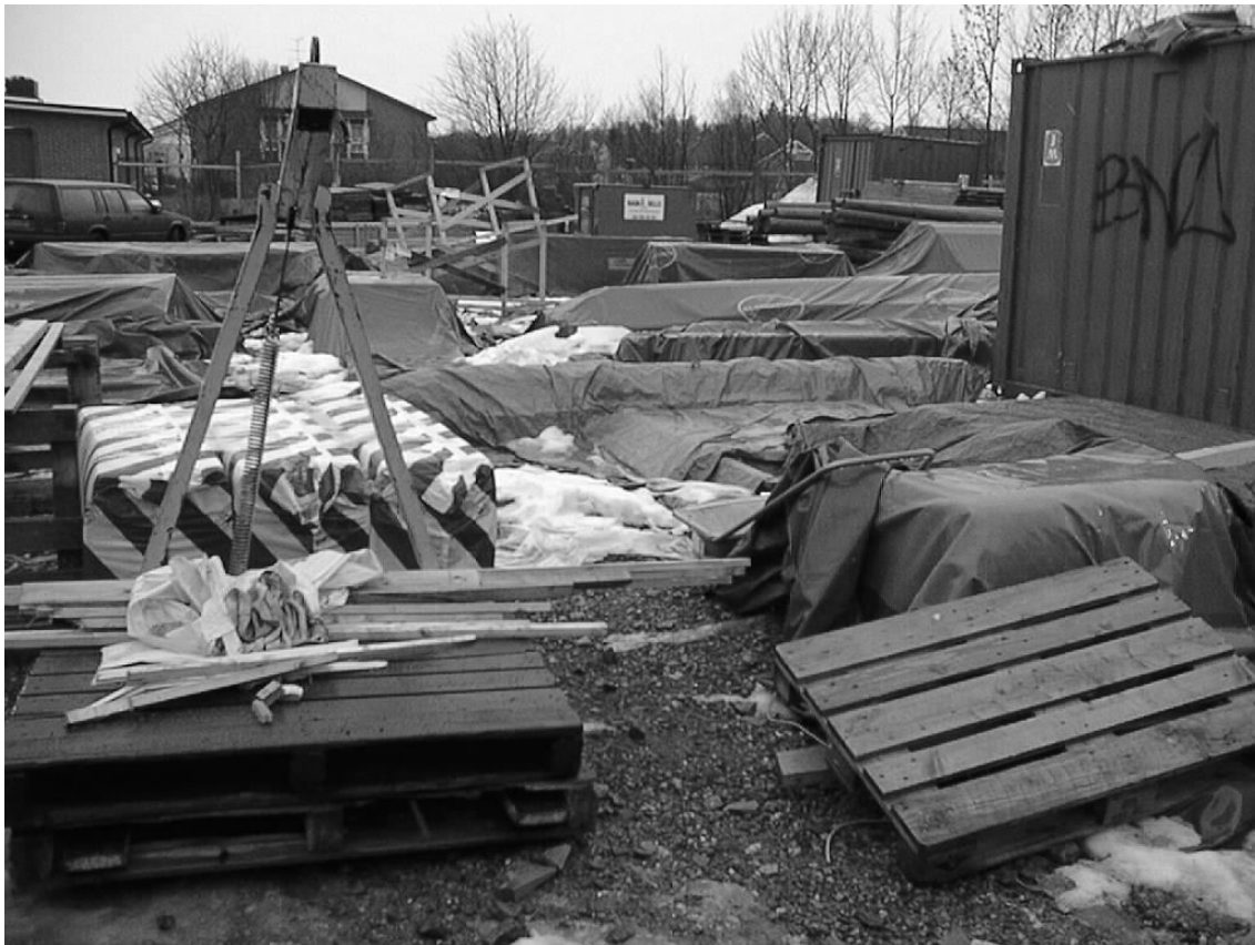
Figure 19: Construction materials on the site.
