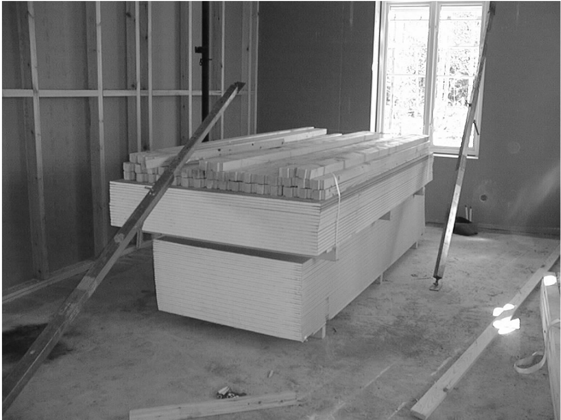
Figure 41: Construction materials unloaded at the place of assembling.
