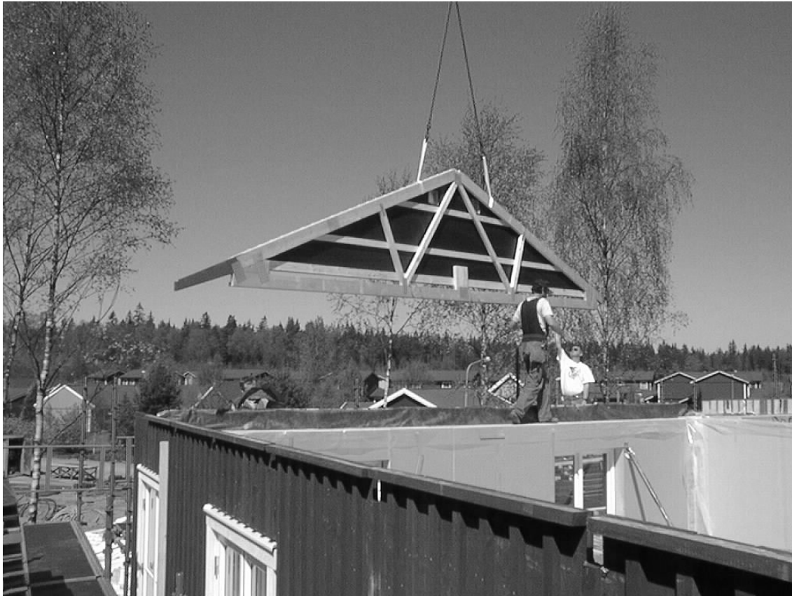
Figure 40: Construction element with attachments to facilitate unloading.
