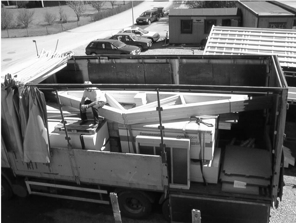
Figure 38: A Just-in-time delivery to a Bo Klok project.
