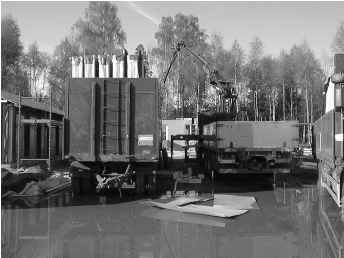
Figure 39: ASG on site performance. Notably difficult site conditions.
