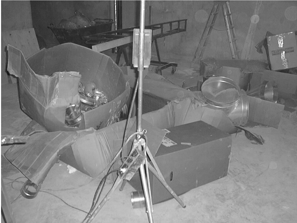
Figure 25: Installation materials on the site.
