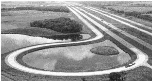
Figure 3.30. The MnRoad research facility (TRB Committee on FS/APT, 2006).
