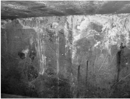
Figure 11. Rust stains and traces of calcium leakage on the side of a prefabricated vertical plate element.
