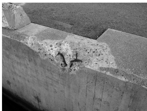
Figure 8. Local damage with corroding reinforcement.
