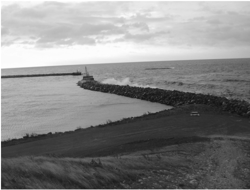
Figure 6. Wave action on breakwaters. Wind direction about 200 degrees.
