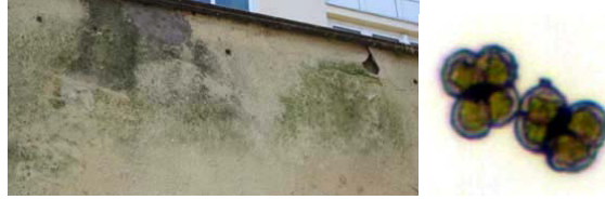
Figure 5.14 Green-algae sp. growing on wall from a façade (“Malen”) in Helsingborg (left) and seen in light microscope (x400) (right)
