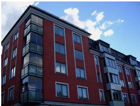
Figure 5.9 Building 2 in Kristianstad with frames of aerated concrete. The red façade is without discolorations
