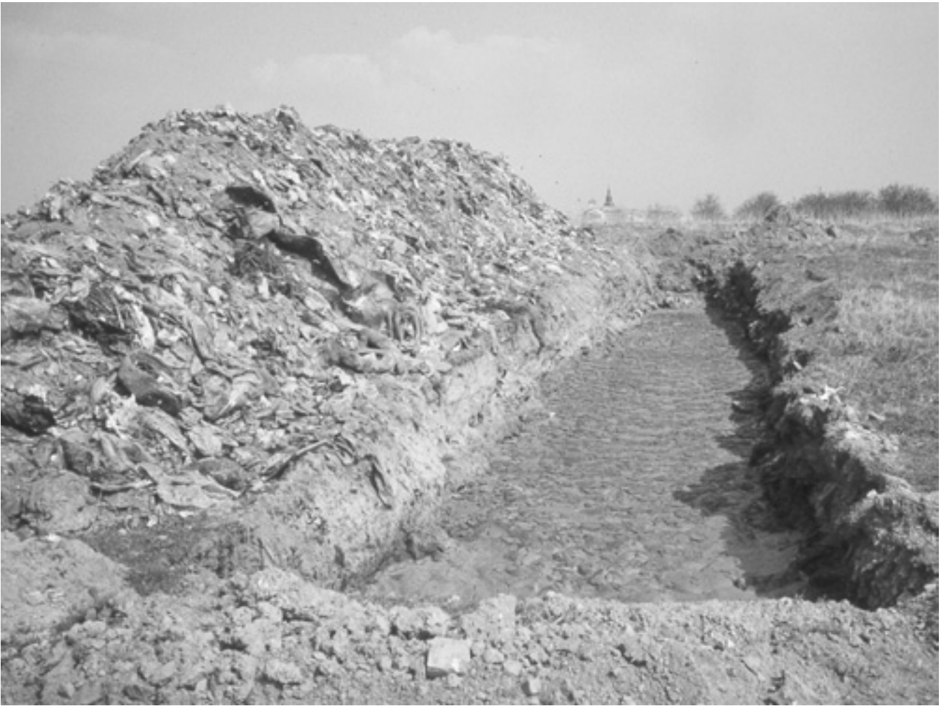
Fig. 2: View of excavated waste material in a trench.
