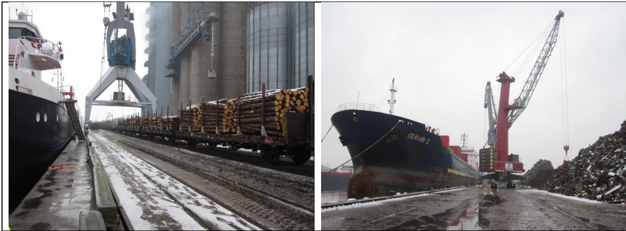
Fig. 1. Examples of vertical loads on quay decks
