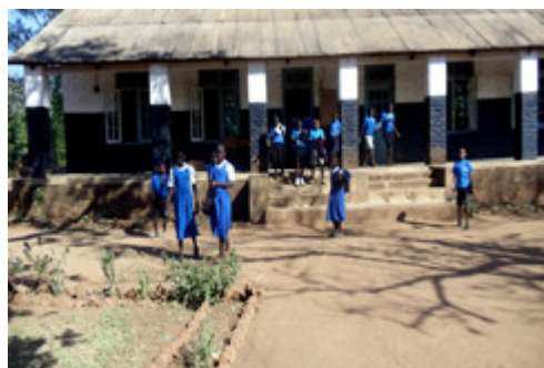
Pic 1. Domasi School steps before intervention.
