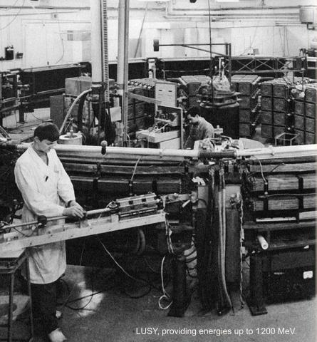
The 35 MeV synchrotron was used for experimental nuclear physics. After a while, there was a need for higher energies to study mesons and other newly discovered particles.
