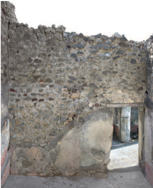
Fig. 25. The South House of Caecilius Iucundus, south wall of the garden room s . Note the collapsed state of the wall, partly sunken into the cellar beneath. By Hans Thorwid.
