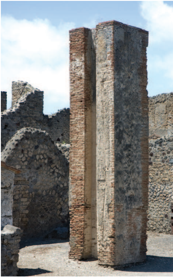
Fig. 13. The second water tower of the Via Vesuvio/Stabiana/Abbondanza line. Note the calcium deposits on the sides of the tower witnessing the overflow from the flooded castellum plumbeum once at the top of the tower. Note also the imprint of pipes along the shaft. By Hans Thorvid.
