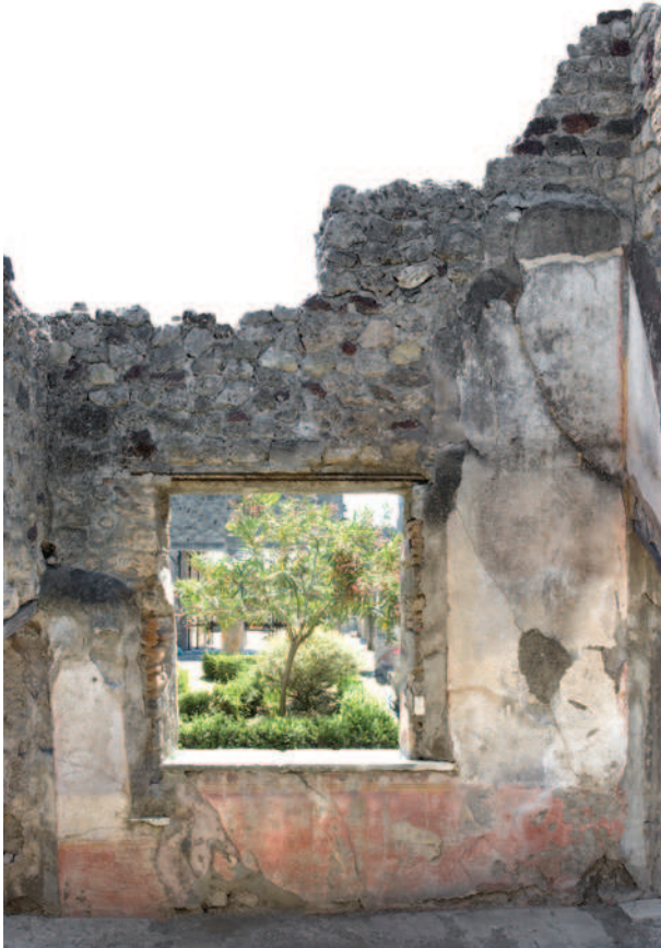
Fig. 26. Window with garden view. West wall of room s of the South House of Caecilius Iucundus. Note the sunken S part of the wall and the broken window-sill. By Hans Thorwid.
