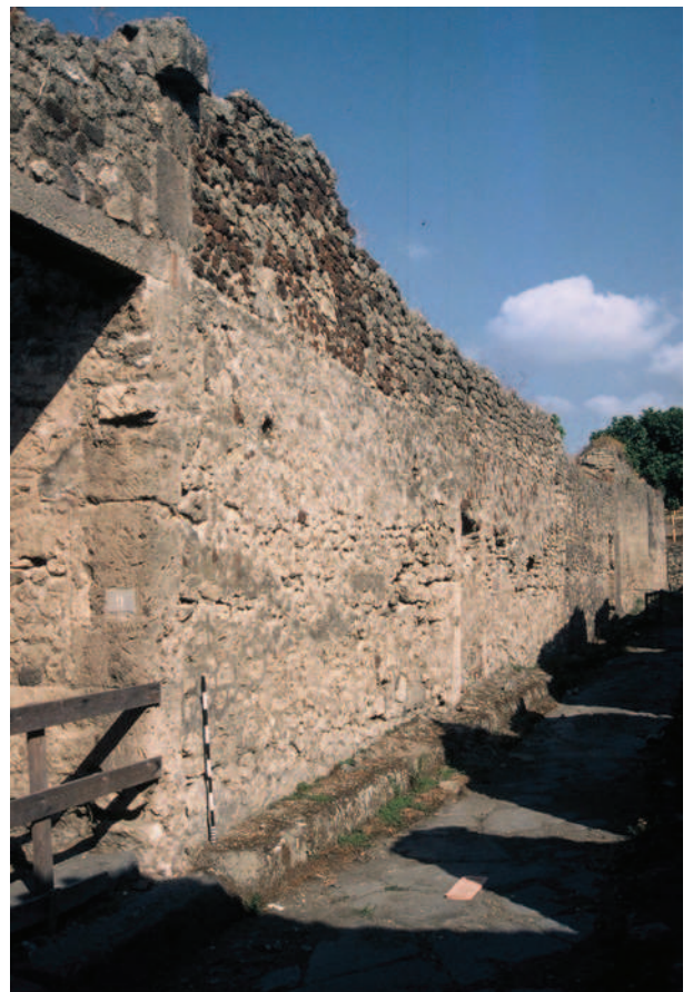
Fig. 4. Vicolo di Caecilius Incundus looking north. The posticum of the Casa del Torello in the foreground. The façades display original rubble masonry. The dark lava incertum of the North House of Caecilius Incundus is easily recognised in between the light masonry used for the façades of the South House and the Casa degli Epigrammi greci. By Arja Karivieri.
