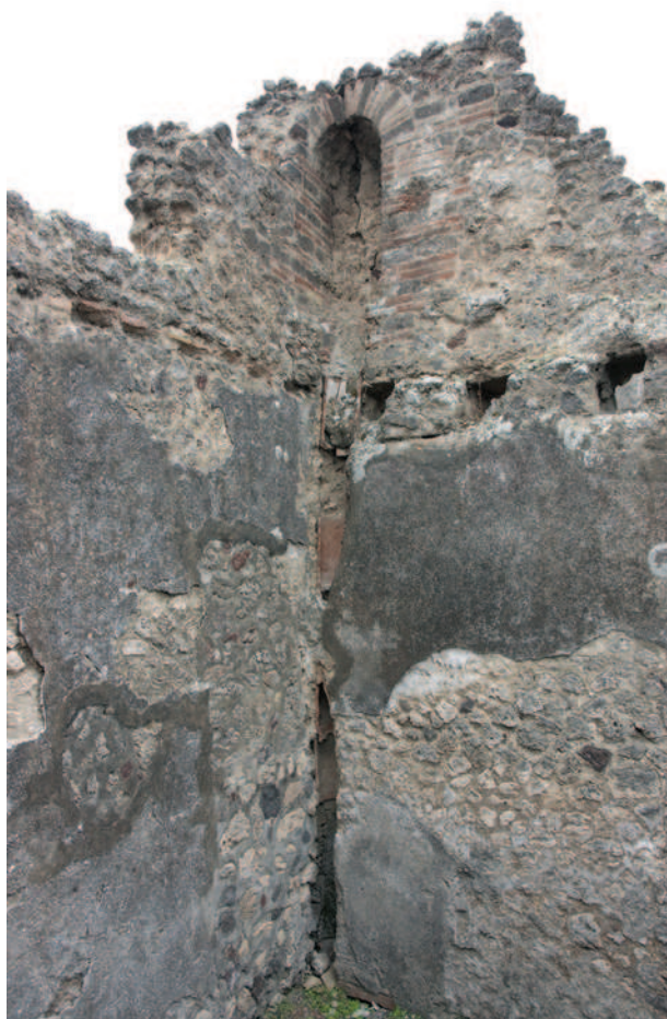
Fig. 31. Rear room of taberna V 1,30 with second-storey privy niche in the SE corner. By Hans Thorvid.
