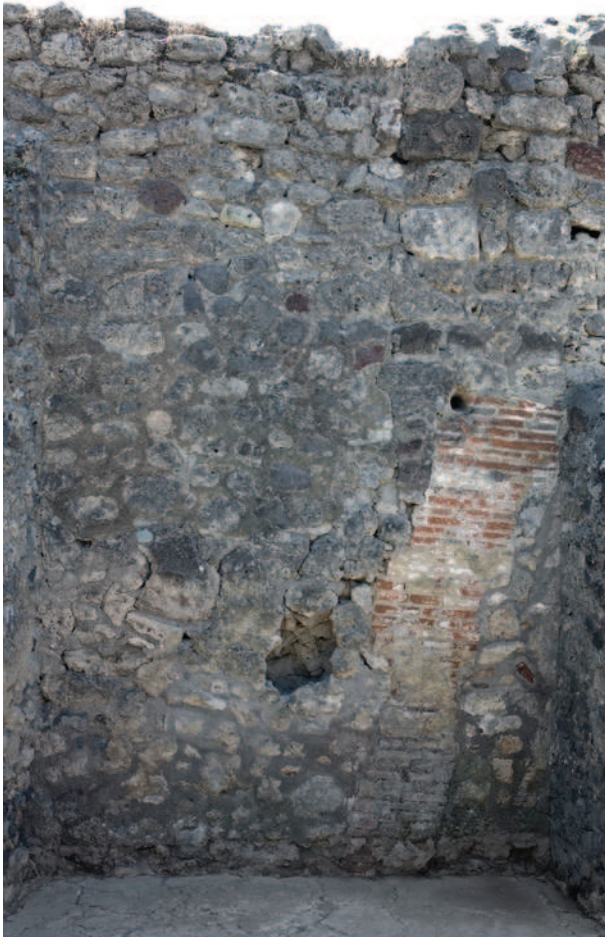
Fig. 23. Brick stitch repairing a fissure in the facing of the south wall belonging to the rear shop (b) of taberna V 1,24. By Hans Thornid.
