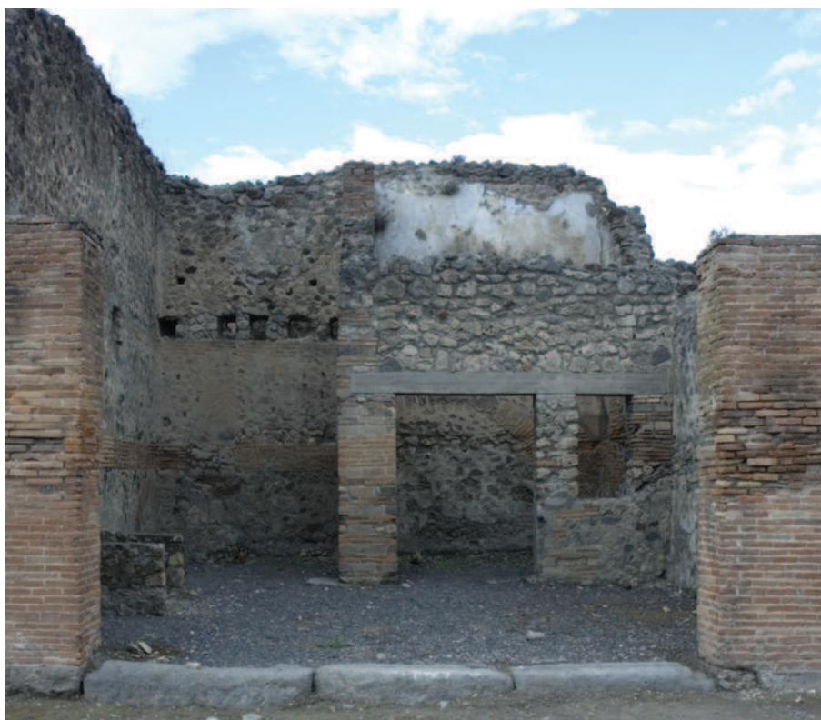
Fig. 18. Taberna V 1,2 on Via di Nola. Note the relieving arch in the rear wall. Note also the damage in the horizontal brick courses further left (W), caused by a post-eruption robber tunnel. By Hans Thorvid.
