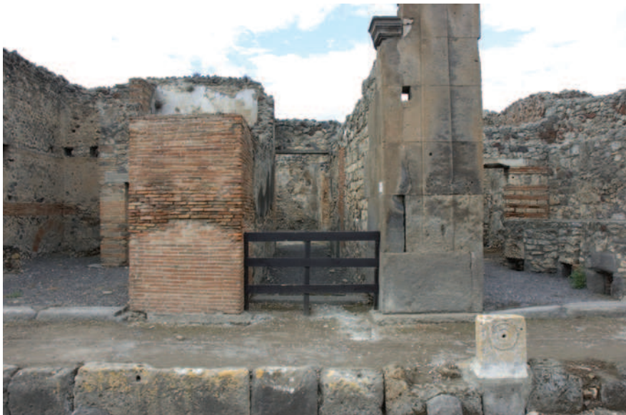
Fig. 8. Entrance of domus V 1,3 and flanking workshops. Note that different masonry is used for the jambs and that both stand on the same kind of foundation. By Hans Thorvid.
