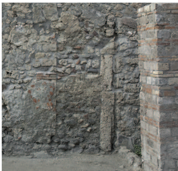
Fig. 38. Detail of Fig. 37: walled-up north doorway of the atrium area of V 1,23, the north House of Caecilius Lucundus . Note the clay lining half way up in the doorway fill and its relation to the plaster (full of pottery sherds) of the north wall proper. By Hans Thorwid.
