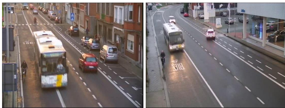
Figure 30 – Observation sites: Kortrijk (left) (3.1 m wide – in line with guidelines) and Ghent (right) (4.2 m wide – not in line with guidelines).
