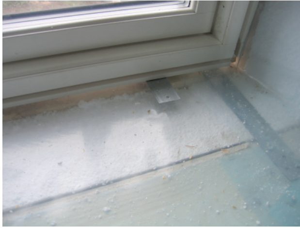
Figure 5.18 Additional metal plates in window opening to be able to mount the windows.
