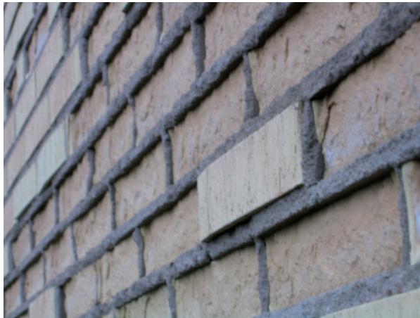
Figure 6.2 Worn out façade brick.
