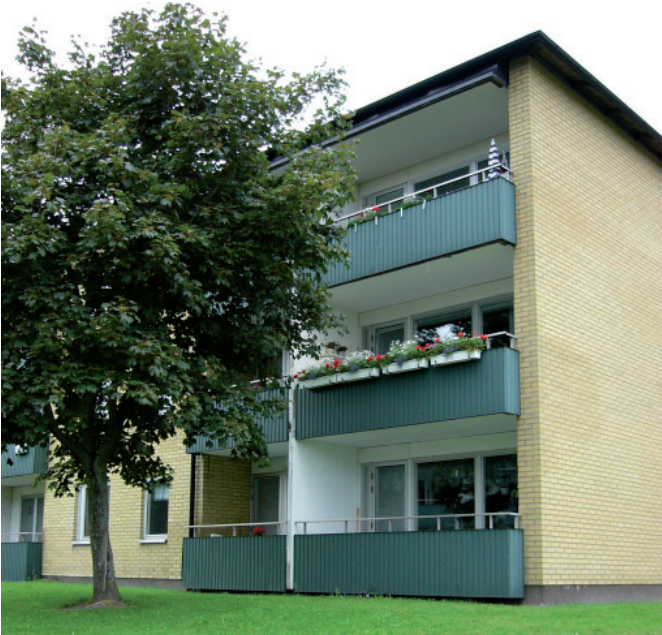
Figure 6.7 Original balcony construction inset into the apartments.
