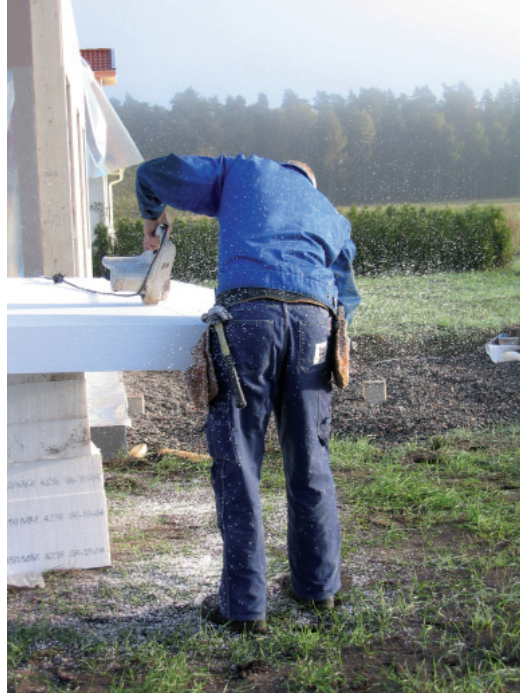
Figure 5.9 Polystyrene sawn up on site.
