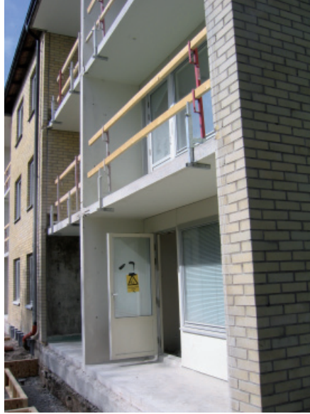
Figure 6.20 Long side walls when the outer part of the existing balconies were sawn off.
