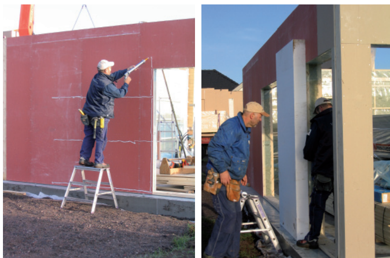
Figure 5.8 Polystyrene glued on the gypsum board.
