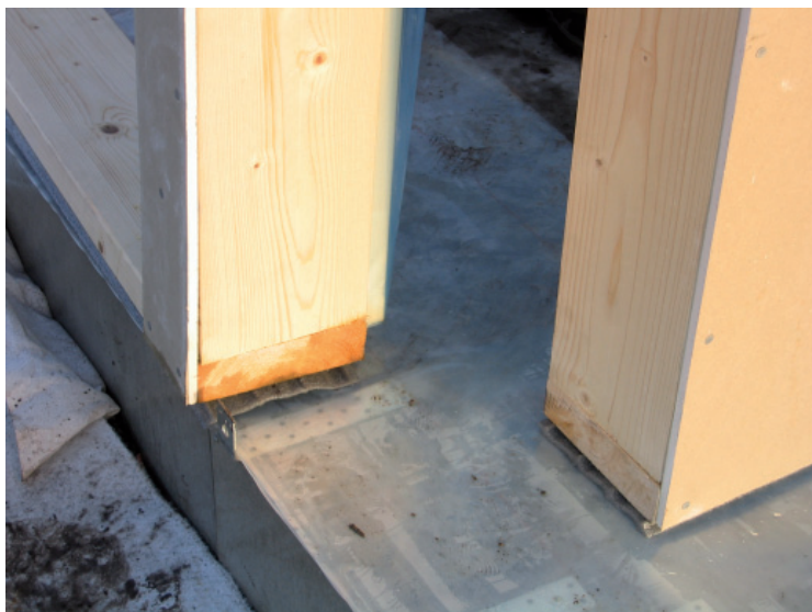
Figure 5.7 Moisture protection of wooden beam construction.
