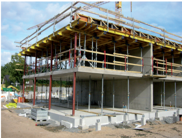
Figure 3.7 Concrete construction cast on site.
