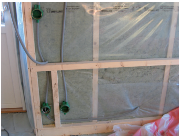
Figure 5.13 Wooden frame construction for installations.
