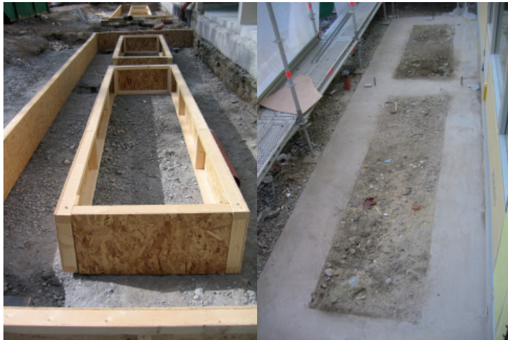
Figure 6.21 Plinths for balconies cast separate from the building construction to avoid thermal bridges.
