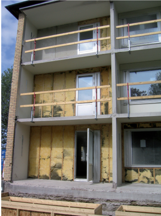
Figure 6.16 Discoloured mineral wool insulation.
