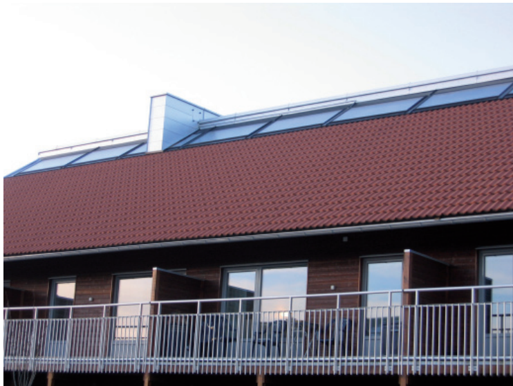
Figure 3.3 Solar collectors.
