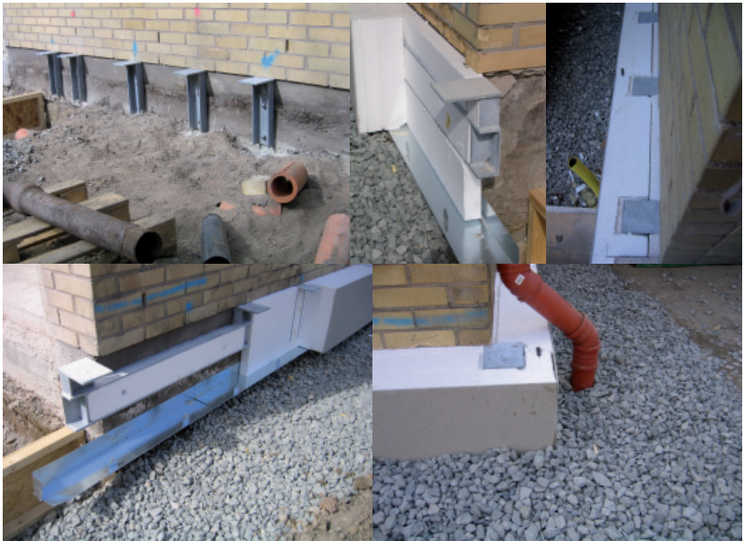
Figure 6.14 Thermal bridge insulation around foundation slab construction.
