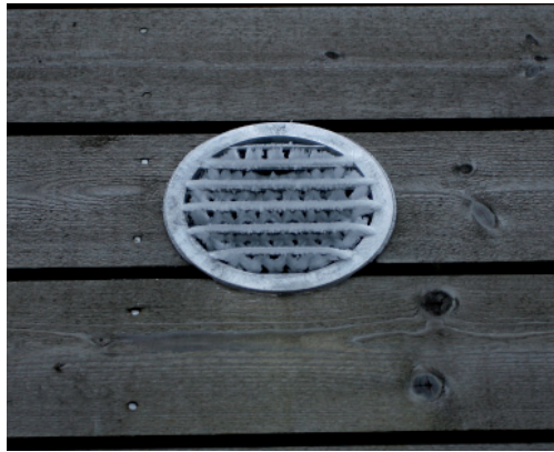
Figure 7.8 Air intake covered by rime.
