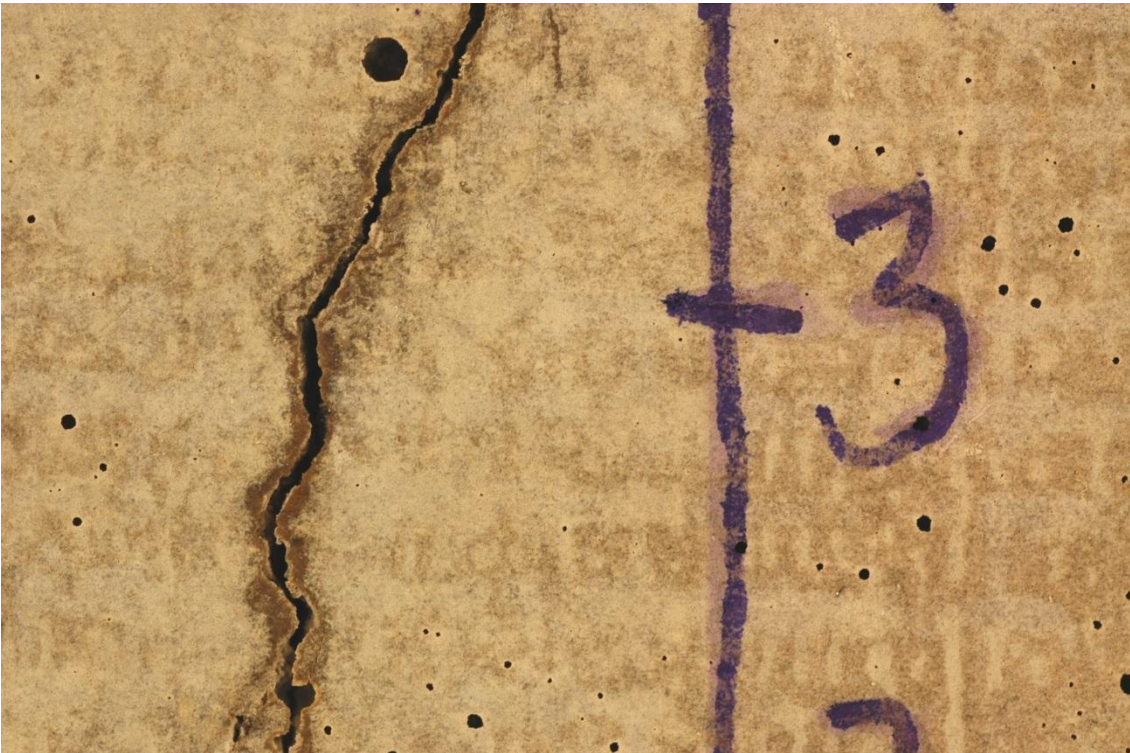
Figure A2.2: 0.4 mm crack after 1 year permanent immersion in sea water. Test series 1, specimen H75-4-1-1.
