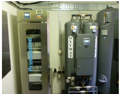
Figure 2 Inside view of the same container. Visible from the left - main PLC, ozone generator, and oxygen generator.
