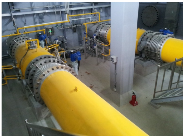
Figure 11 A full-scale installation of static mixers in the main flow pipes in a potable water plant in South Korea. Photo by PAOR CO., Ltd. (reproduced with permission).
