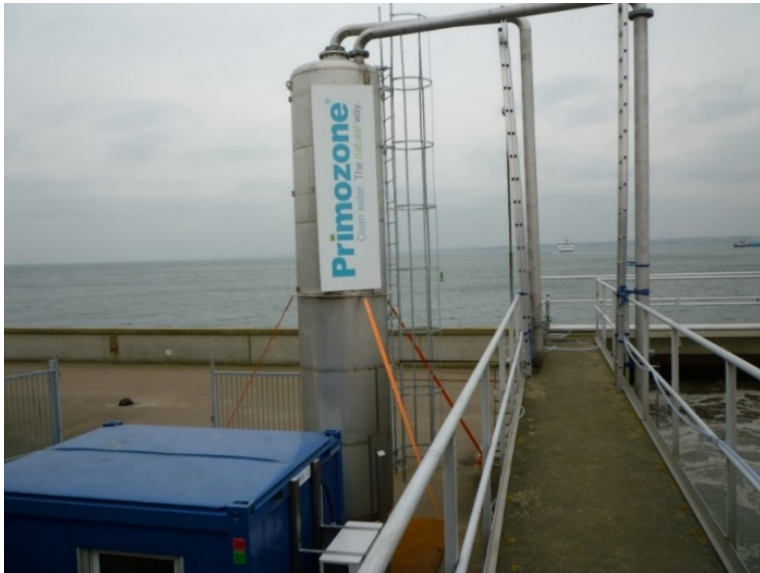
Figure 4 Picture of the container and pressurized reaction vessel installed at Öresundsverket WWTP.
