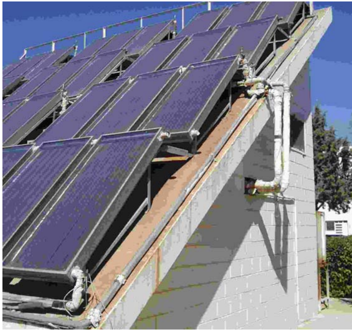
Fig. 4.1.8 Photo of the existing large system flat plate collectors at the RSS.
