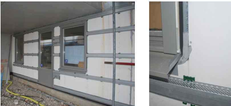
Figure 4. Arrangement of horizontal, vented metal supports with depth 25 mm (left) and a close up which shows the web perforation (right). The function of the green plastic spacers behind the supports is to level out unevenness in the substrate.
