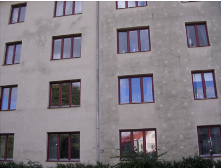
Figure 2.7: A façade that shows white spots.
