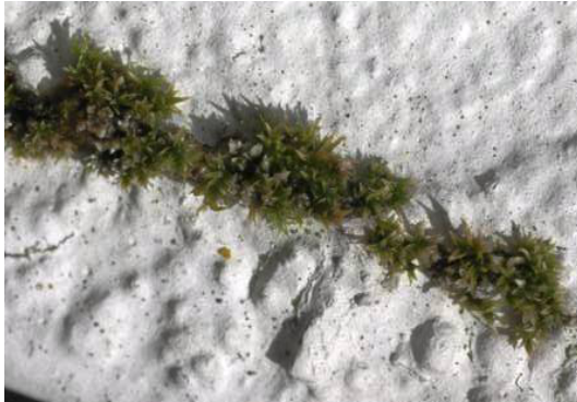
Figure 3.6: A moss growing in a crack between the render and a plastic shell from a specimen used in the investigation of Paper IV.
