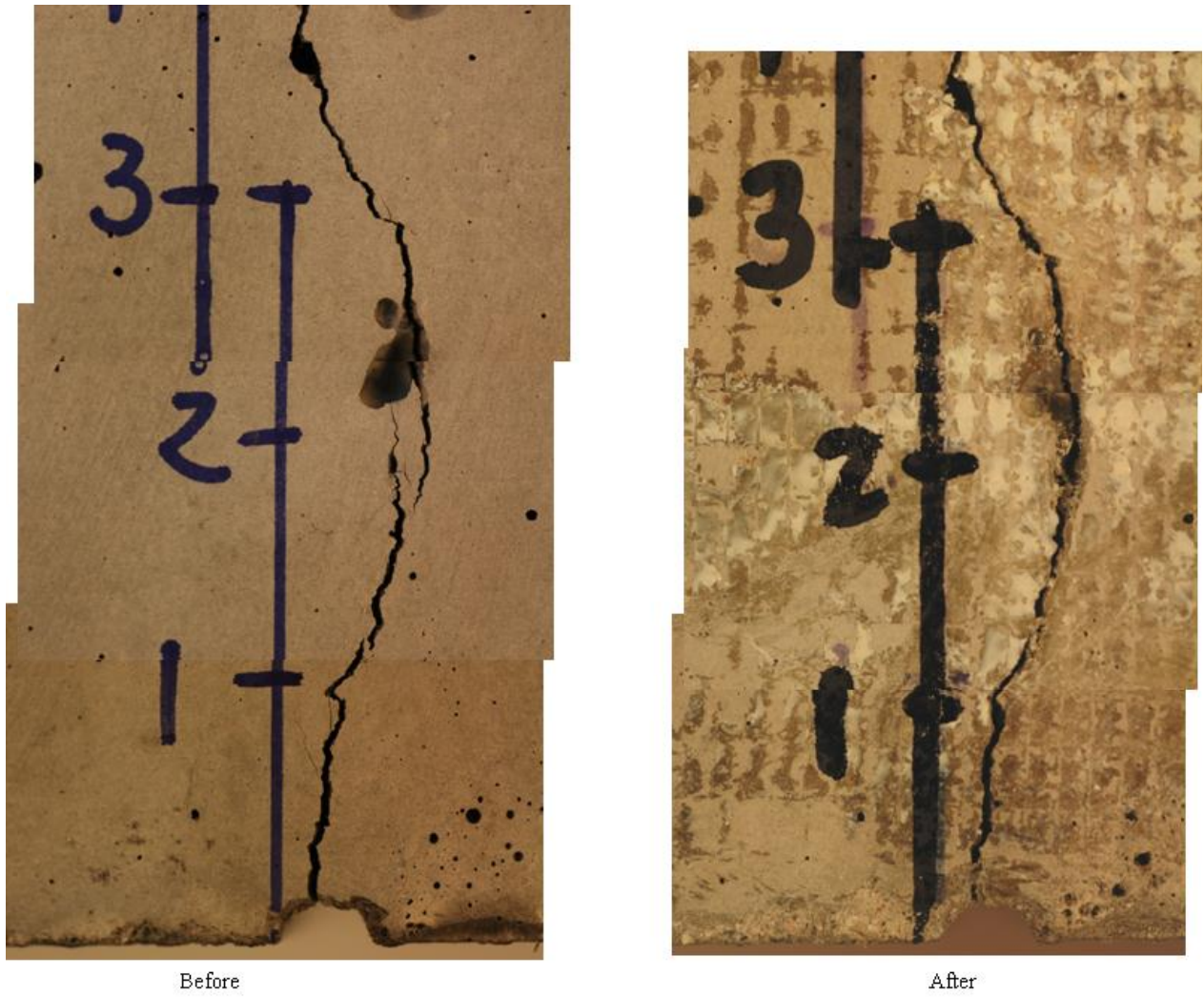
Figure A1.12: Water suction from the un-cracked side. Crack width 0.4 mm. Cover 55 mm. Specimen H55-4-3-2
